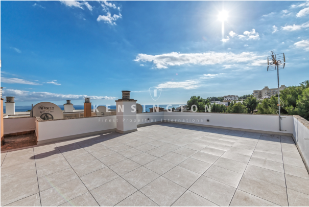
Upper rooftop terrace
