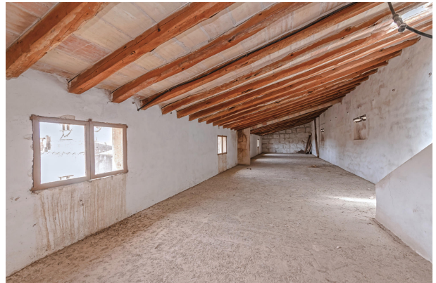
New wing (attic)
